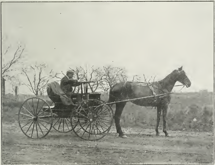
FILLING IN THE ROADS BETWEEN CONTROL LINES
